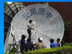
FY-2H DB Station Installation in Bangladesh
