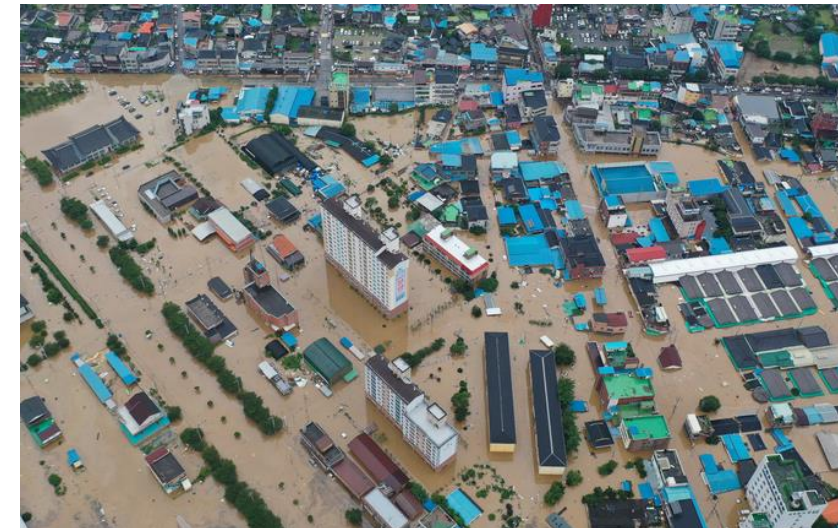
Flooding in residential area, Aug. 10, 2020
